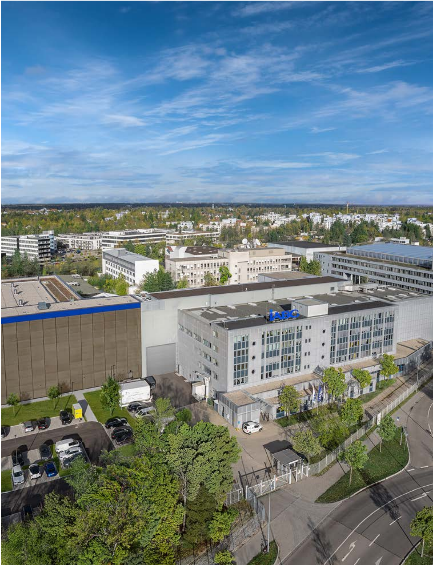
IABG Space Centre, Munich, Germany, since 1965
