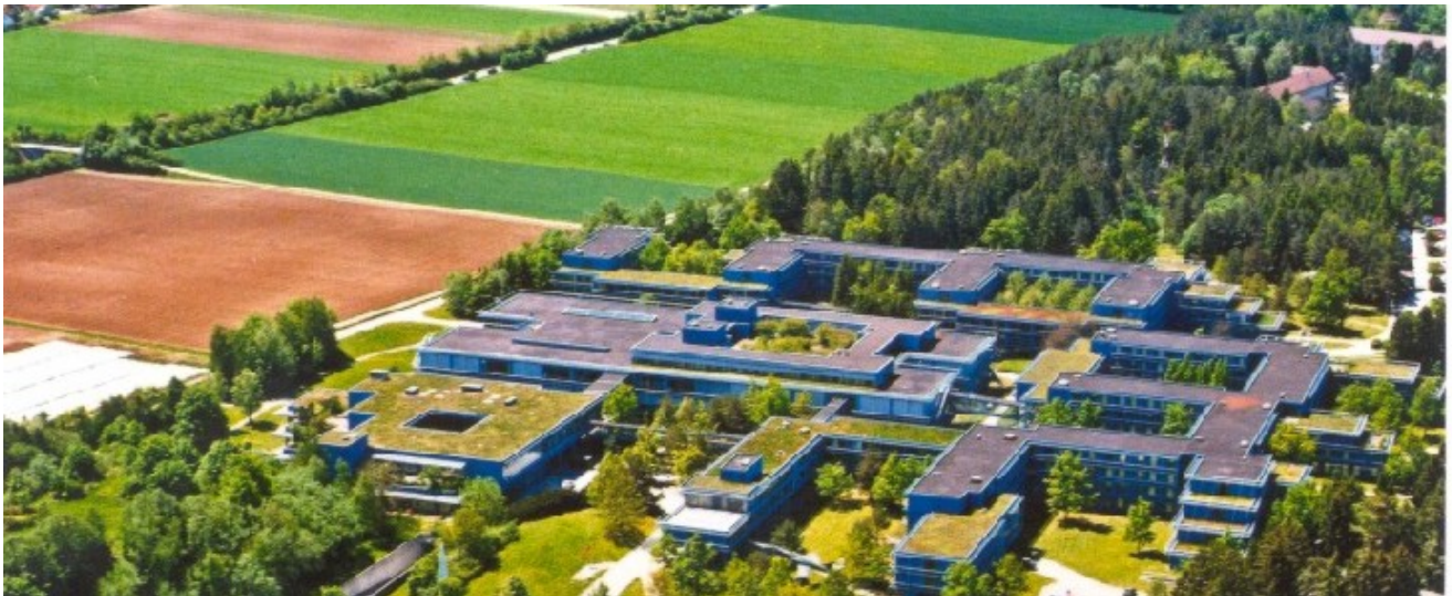
The "Blue Palace" - School Building and Accommodation Quarters
